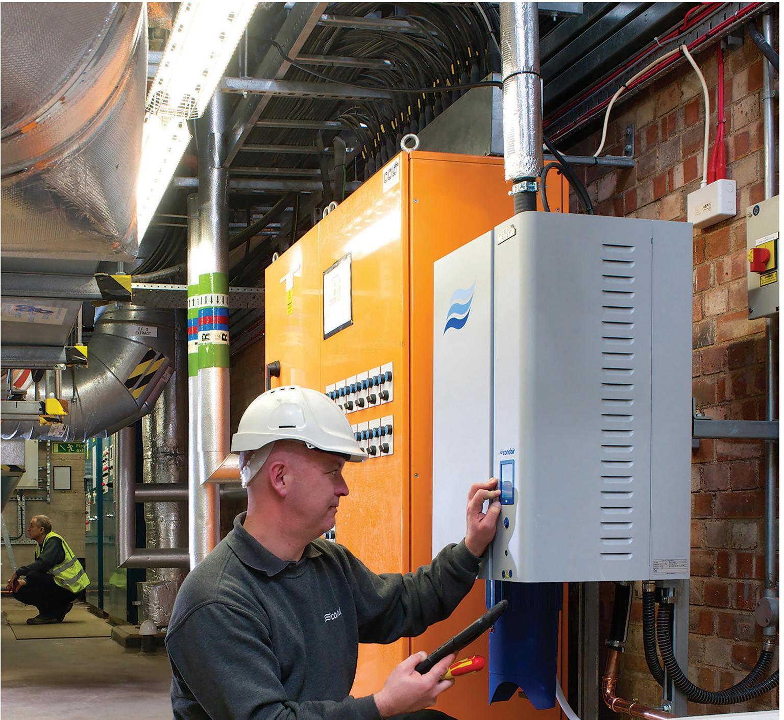
The most common humidifier any HVAC contractor is going to come across is a self-generating, electric steam humidifier. These will typically provide steam to an air handling unit but are also available for direct room humidification with a fan unit. However, for the sake of this guide, I'm going to focus on AHU humidification, as this is the most common.
